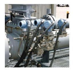
SRE directly relates to flow measurement error and therefore a very important topic to those who buy and sell natural gas. This paper will focus on methods to measure and quantify Square Root Error and subsequent Gauge Line Error, while also recommending several techniques to reduce pulsation effects on natural gas measurement.
