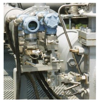
**Figure 10:** Parker's Direct Mount System. The manifold system reduces effect of Gauge Line Error on the total measurement system. Note the reduced numbe of leak points and sensing line length, and uniform diameter between the orifice ports and the measuring elements.
