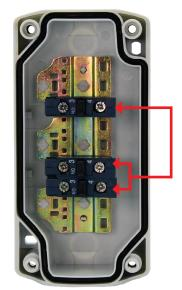
The switch terminal blocks are located inside the back of the control station enclosure.
